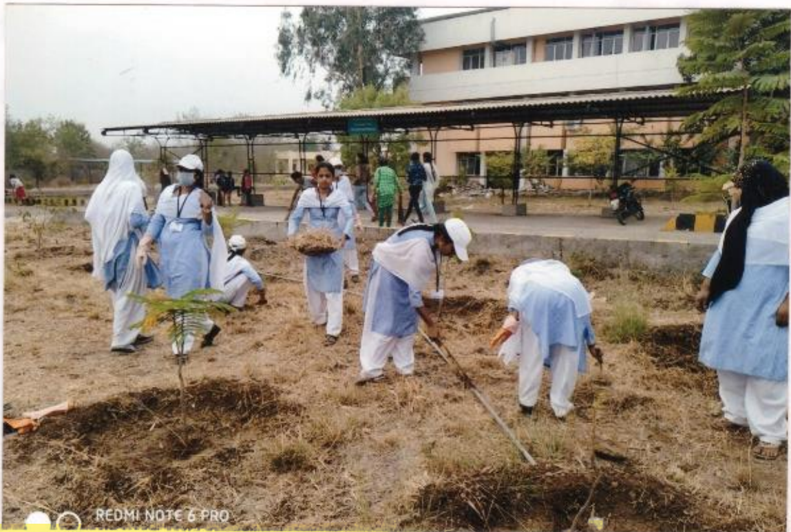
Digging Ground for Tree Plantation in P. A. H. Solapur University, Solapur
